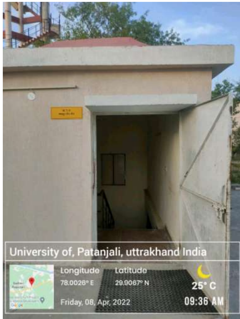
Sewage Treatment Plant at the University of Patanjali
