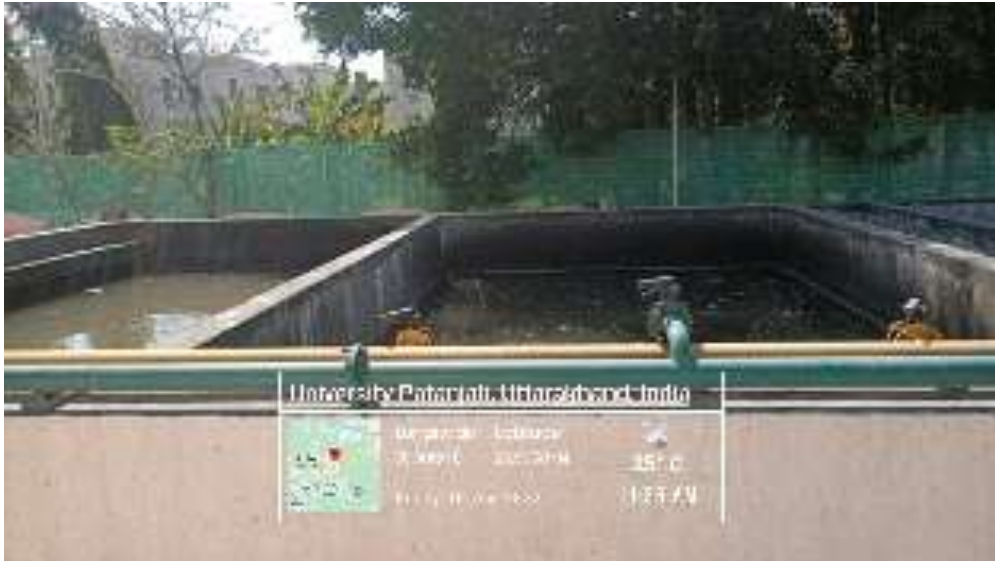
Sewage water in process
